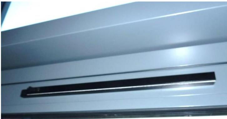
Figure 6. Trickle vent closed (Source: MEARU)
