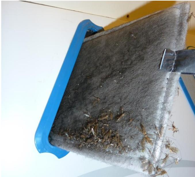
Figure 7. Inadequately maintained filters (Source: MEARU)
