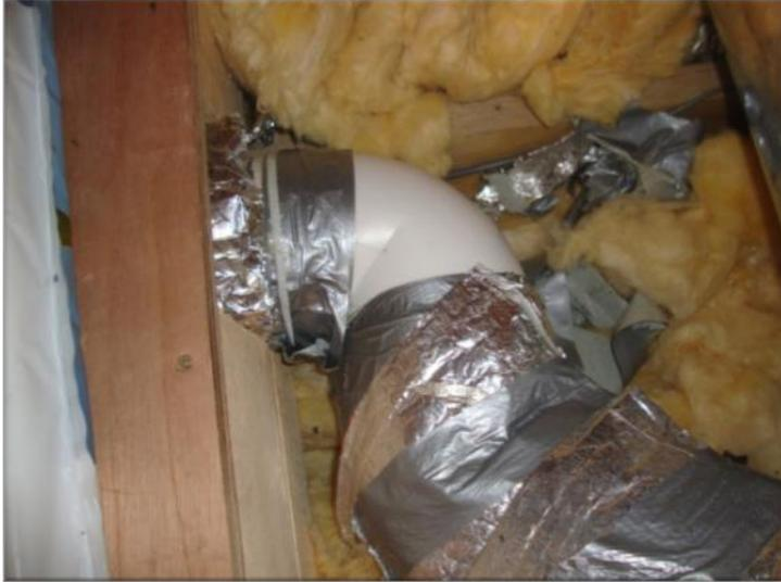
Figure 5. Duct bend un-insulated in cold roof (Source: Eco-Energy NI)
