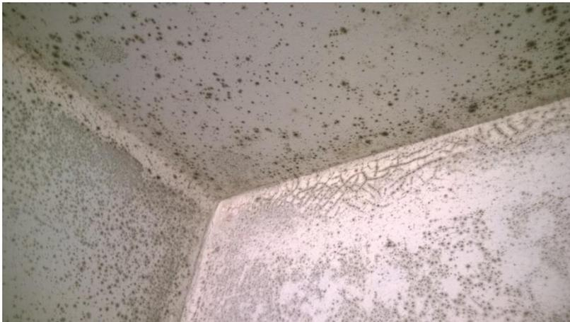
Figure 1. Mould growth on the ceiling of a poorly ventilated bathroom (Source: MEARU – Mackintosh Environmental Research Unit, Glasgow School of Art)
